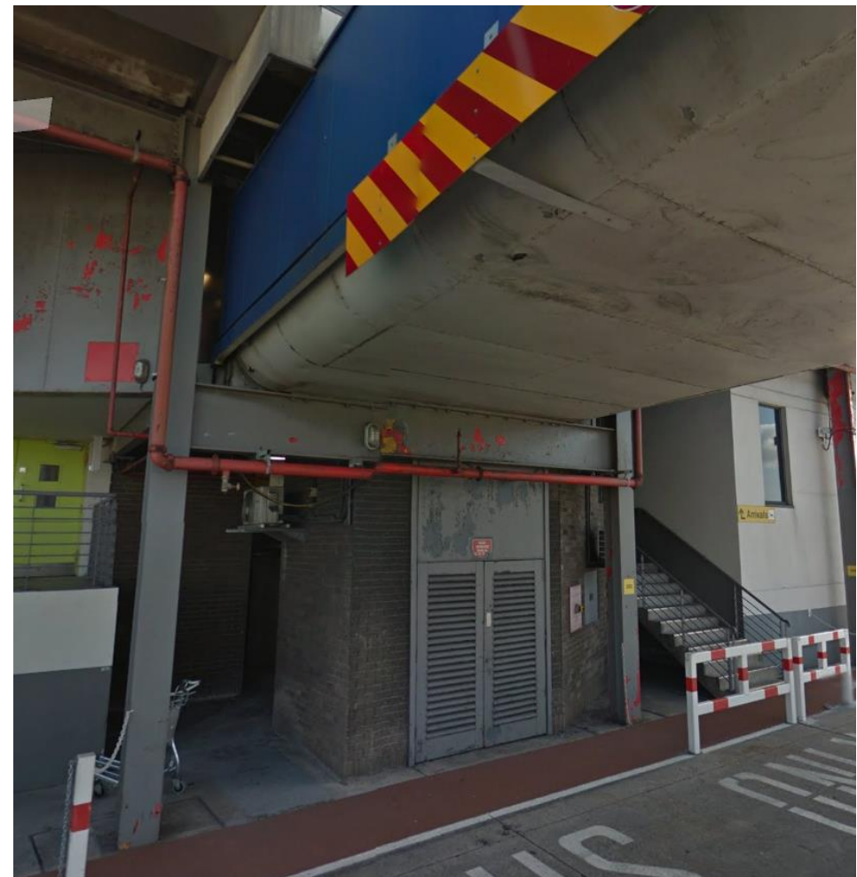
Figure 3-9 - Existing Fixed Link Connection to Pavilion at Level L15
