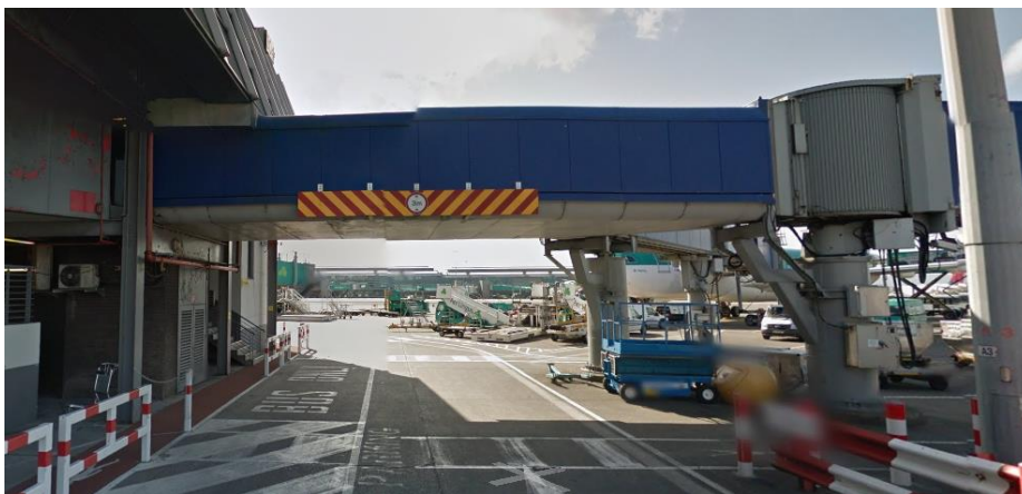
Figure 3-8 - Existing Fixed Link Connection to Pavilion at Level L15
