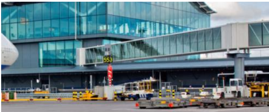
Figure 3-6 - Example Prefabricated Fixed Link and Support Column
