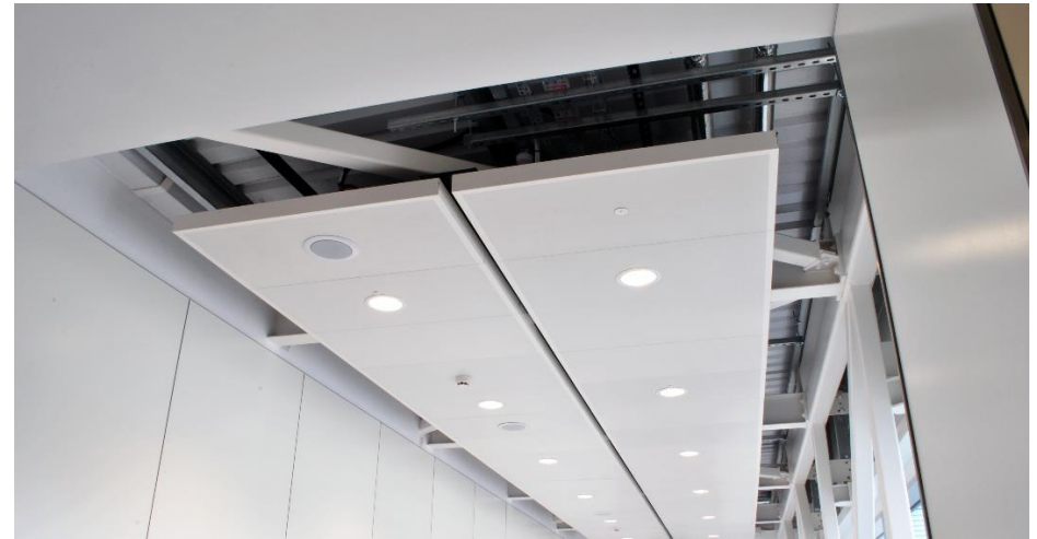
Figure 2-18 - Proposed suspended ceiling system with integrated lighting
