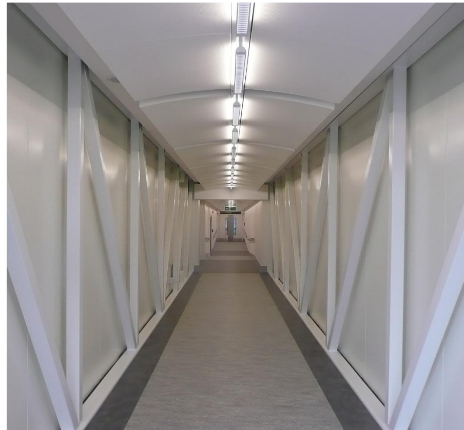
Figure 2-16 - The fixed links will be modular prefabricated structures with exposed steel on the inside and durable finishes to the floors and walls.
