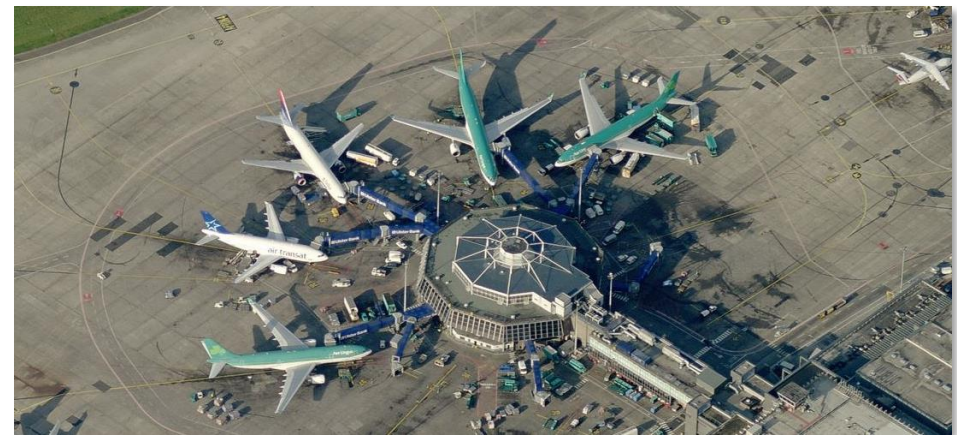
Figure 1-5 - Existing Pier 3 decagon and surrounding aircraft stands
